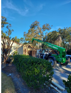
Trusses going up on for garage roof.
