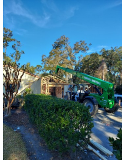
Trusses going up on for garage roof. ←
